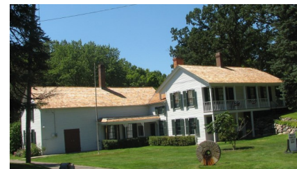
NEW roof Installed back in 2010
